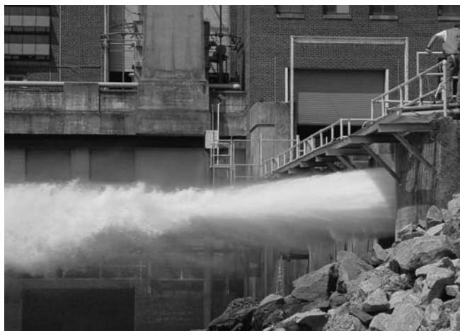
In October 2005, the new Pratt fixed cone valve at South Carolina Electric & Gas Company's Saluda hydro facility/McMeekin coal-fired generating station complex released 113,000 gallons per minute for nine continuous days.
