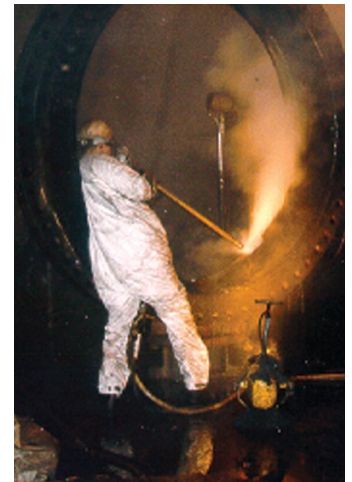
HIGH PRESSURE STEAM CLEANING OF THE VALVE BODY.
