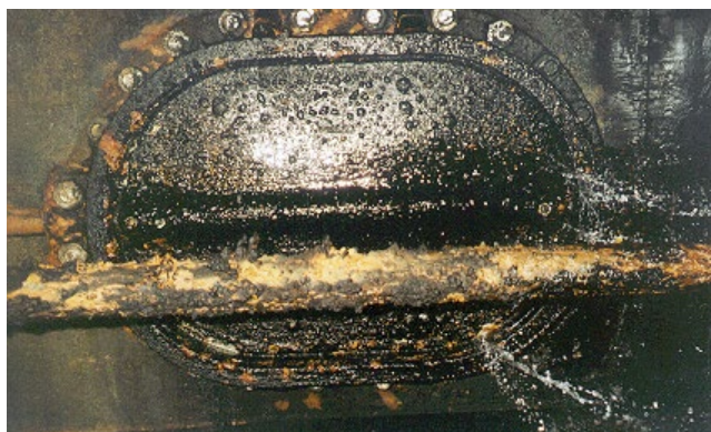
PRIOR TO REPLACEMENT 24" BY 36" OBROUND VALVE
