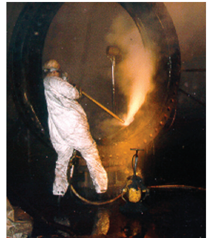
High pressure steam cleaning of the valve body.
