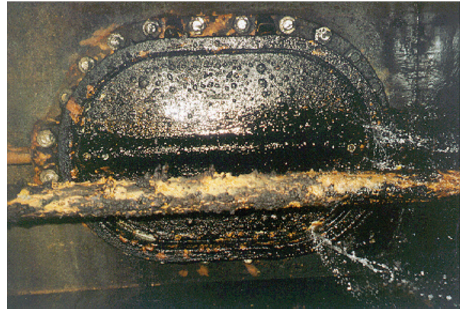
Prior to Replacement 24" by 36" Obround Valve
