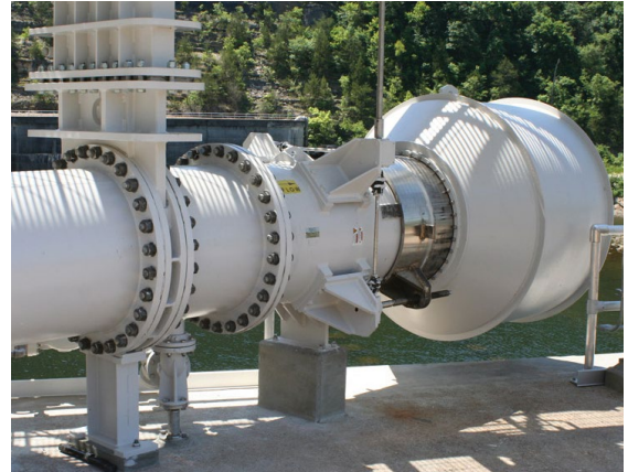
30" FIXED CONE VALVE WITH HOOD
