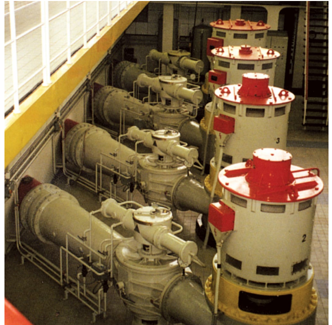
24" ROTARY CONE VALVES IN OPERATION SINCE 1956.
