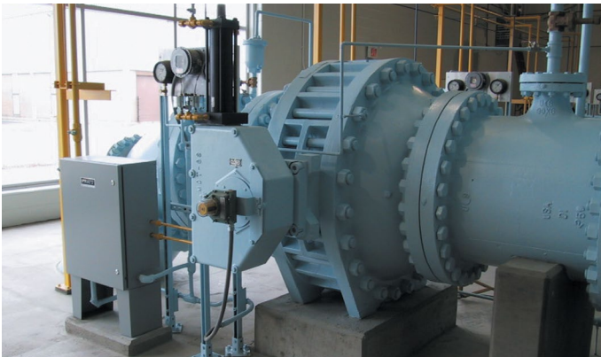
RUBBER SEATED BALL VALVE INSTALLATION
