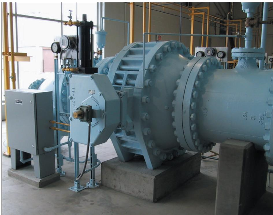
Rubber Seated Ball Valve Installation
