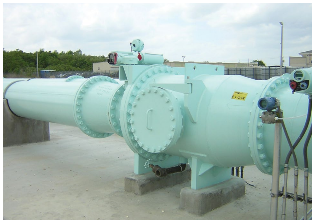
36" Model 711 Inline Sleeve Valve
